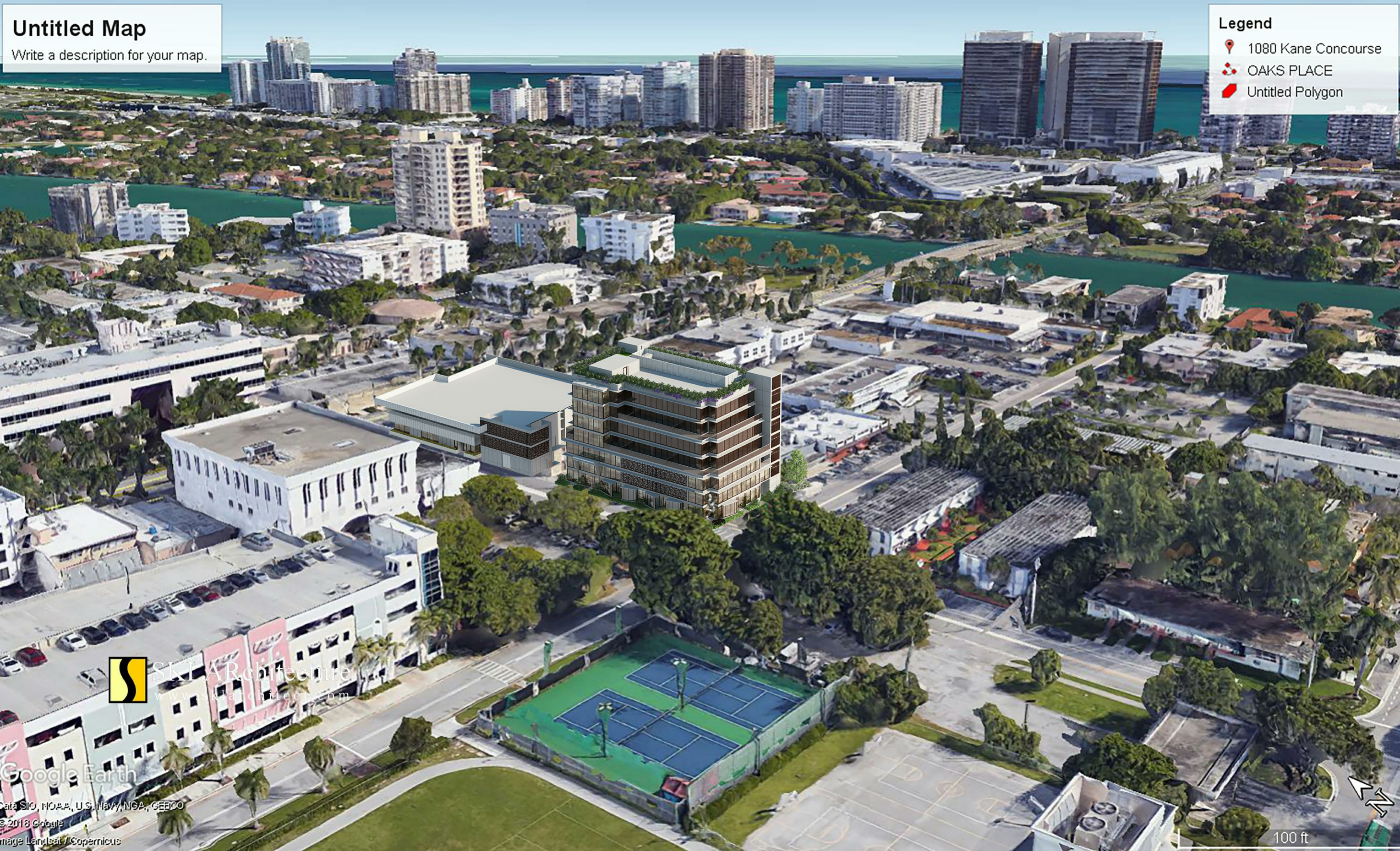
SOUTH WEST AERIAL VIEW
