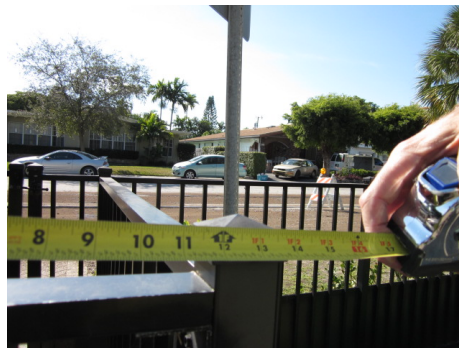
Gate offset less than 18 inches
