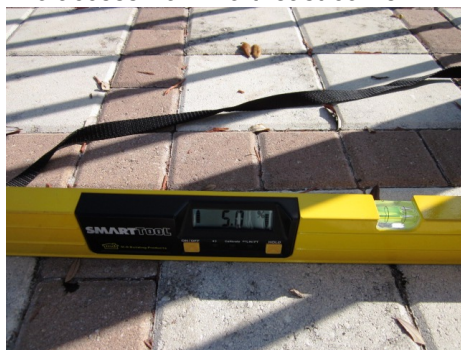
Running slope at NW gate 5%
