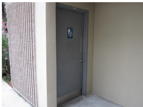
Entrance door sing on door
