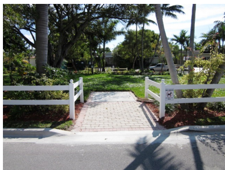
Curb ramp provided
