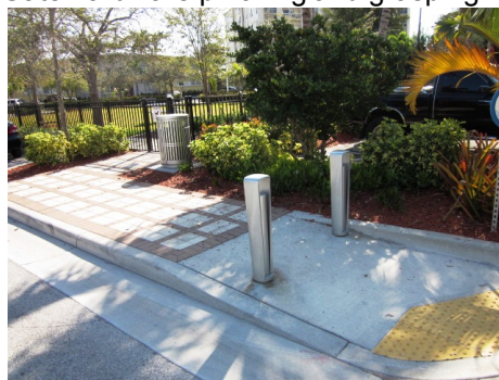
Cross slope NW curb ramp 4%
