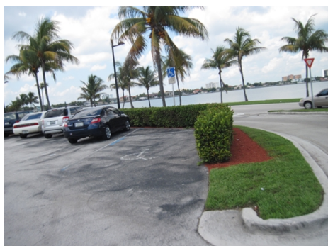
No access aisle No access aisle
