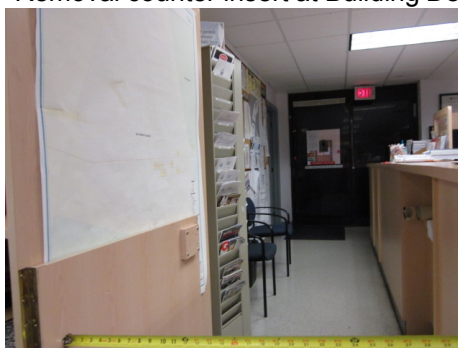
Gate to offices less than 32 inches clear
