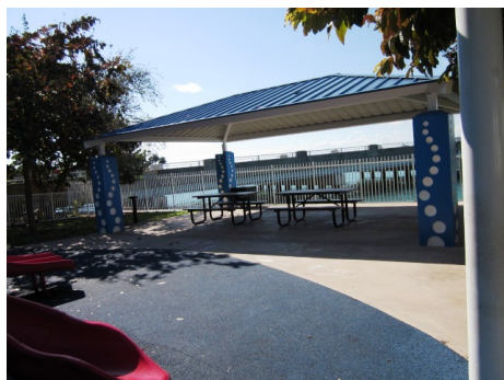
Picnic tables not accessible
