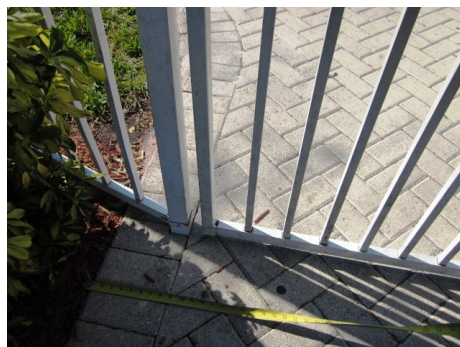
Offset pull side of gate
