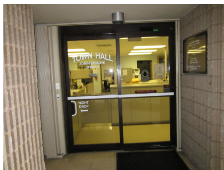
Automatic doors at Clerks Office
