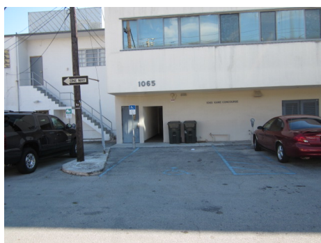
Accessible parking provided 1065
