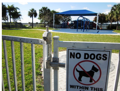
Gate hardware not accessible
