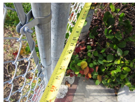
North gate offset pull side 12 inches
