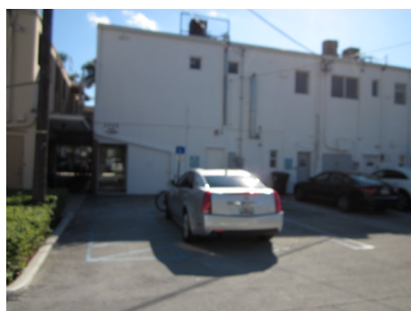
Accessible parking provided 1025
