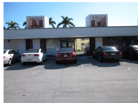
Accessible parking provided 1065
