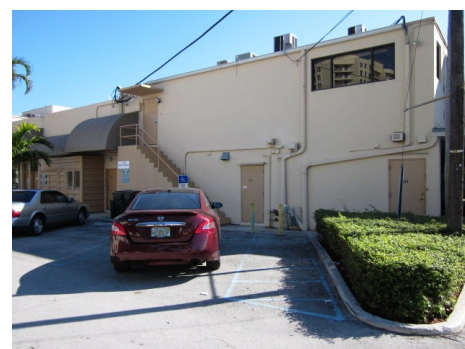
Accessible parking provided 1021
