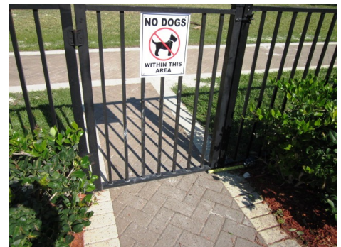
Gate offset less than 18 inches
