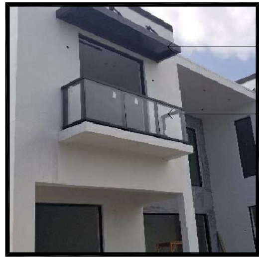
BALCONY GLASS RAILS AND ALUMINUM CANOPIES
