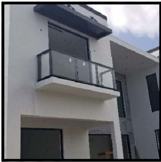
BALCONY GLASS RAILS AND ALUMINUM CANOPIES
