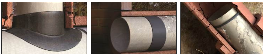
Fig 4. Pipe Renewed by CIPP
