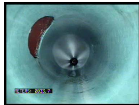
Fig 2. Pipe Renewed by CIPP
