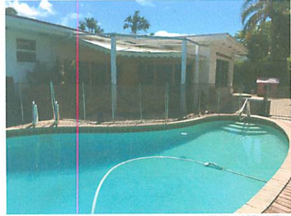
REAR NORTH VIEW
