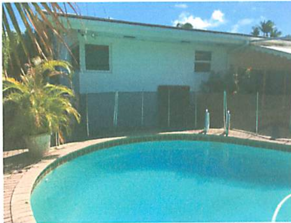
REAR NORTH VIEW
