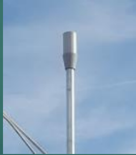
Existing JEA Streetlight Pole
