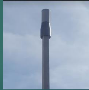
New Concrete Pole
