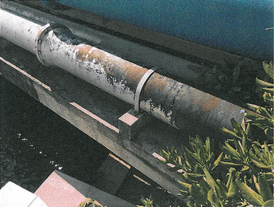
SEWER LINE AND SUPPORT NEAR WEST CONNECTION
