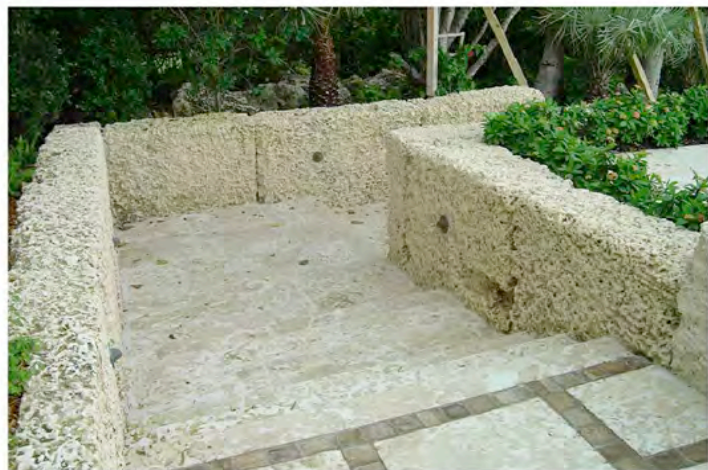
Random size Keystone slabs set on concrete base with 4" granite joint infill
