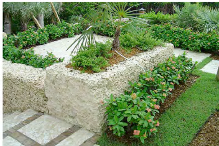
Random size Keystone slabs set on concrete base with 4" granite joint infill
