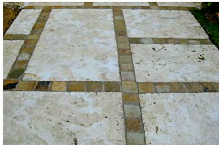
Random size Keystone slabs set on concrete base with 4" granite joint infill
