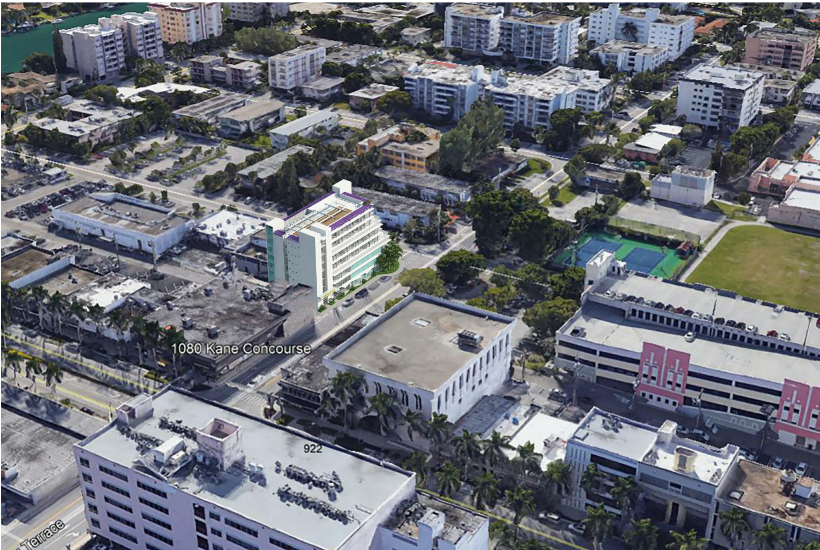
SOUTH EAST AERIAL VIEW
