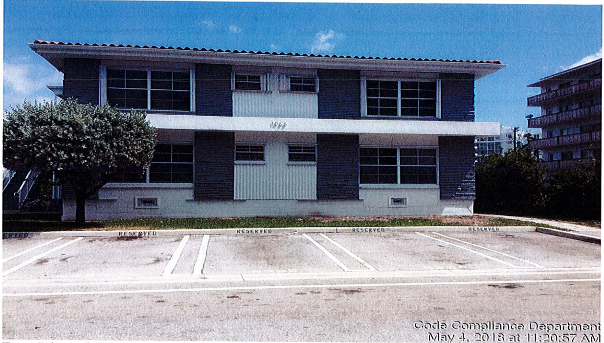
Front View of the property- Tree removed and not replaced.
