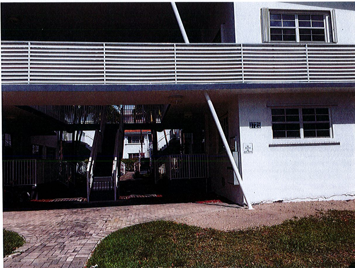
9725Electrical2.JPG Electrical Inspection TDR May 03, 2018
