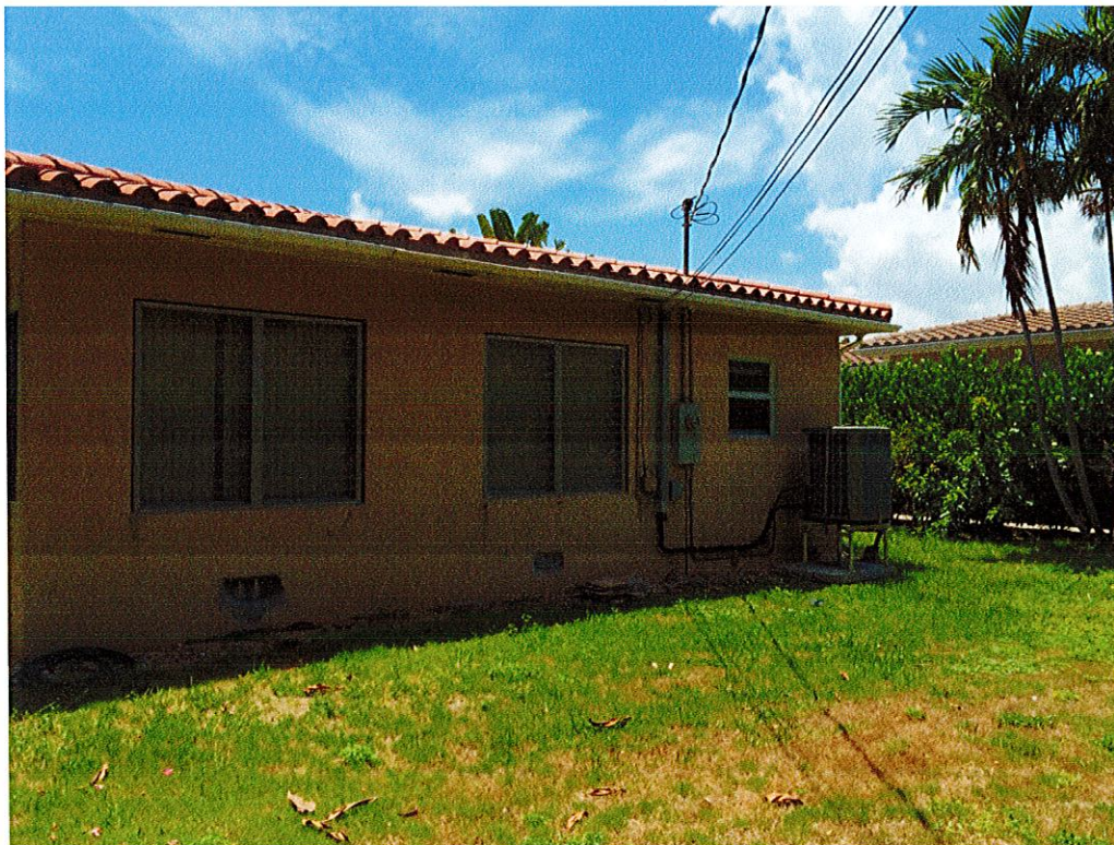
EXISTING SITE -REAR SIDE VIEW
