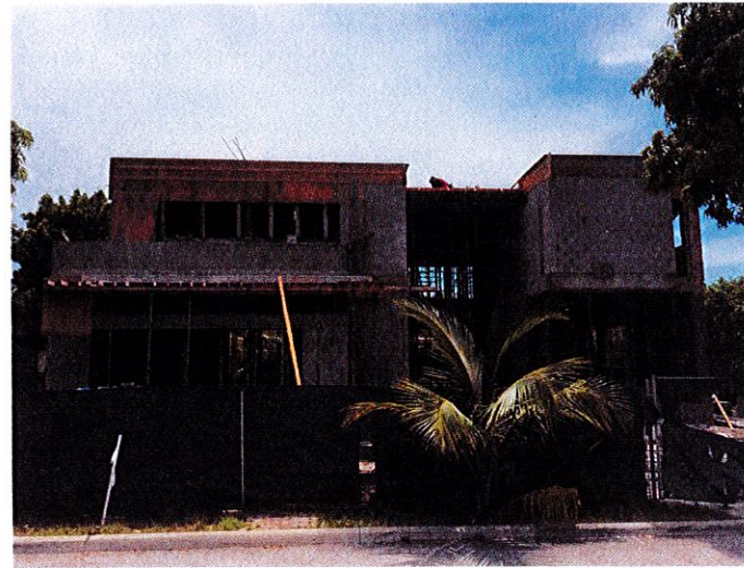
UNDER CONSTRUCTION TO THE EAST
