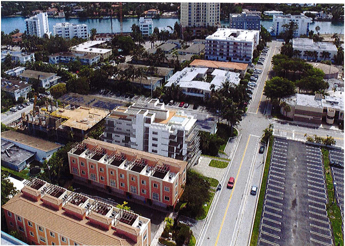
2 S.W. AERIAL VIEW
