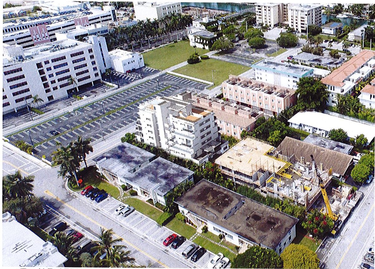
1 N.E. AERIAL VIEW
