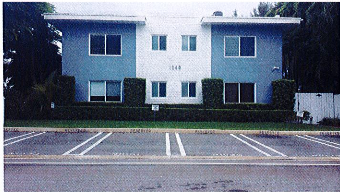
ADJACENT EAST NEIGHBOR
