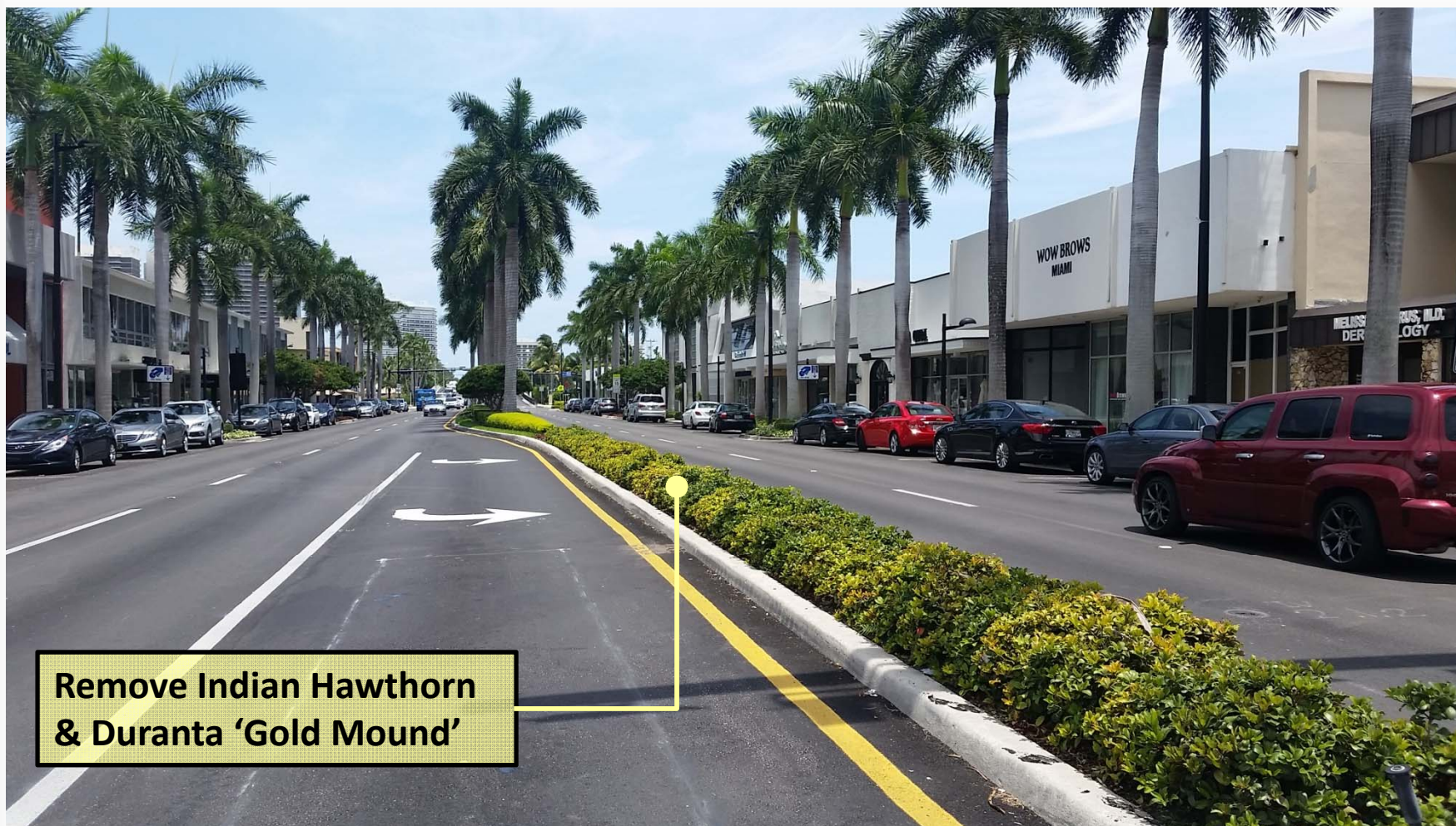
Existing condition looking East at Bay Harbor Terrace
