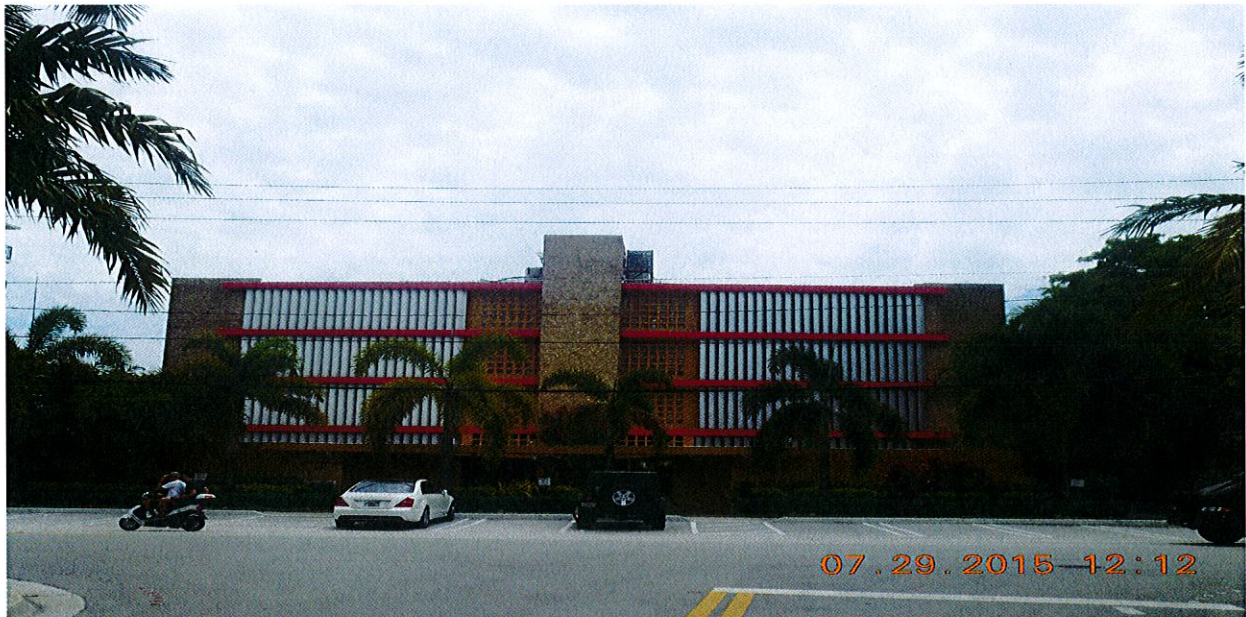
Front view- No violations observed.
