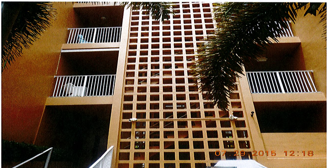
Stairwell view- No violations observed.
