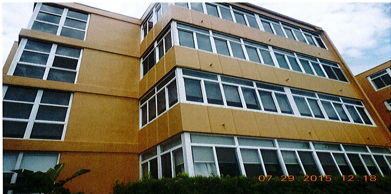
Rear view- No violations observed.
