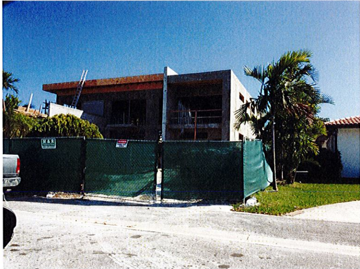
VIEW - CONSTRUCTION TWO LOTS DOWN FROM 1310 95TH STREET
