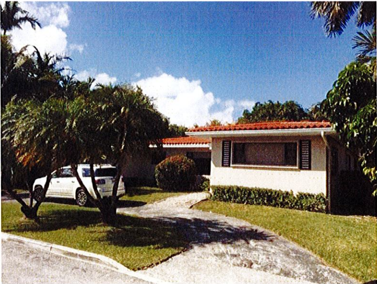
SITE CONTEXT VIEW - 1311 95TH STREET
