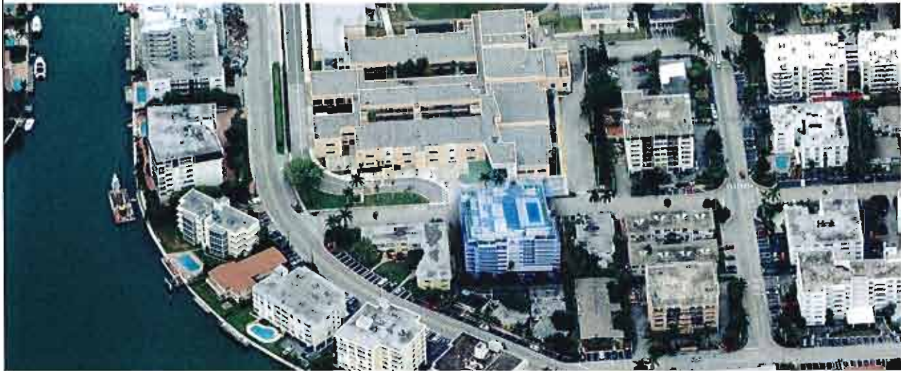
AERIAL VIEW FROM SOUTHWEST
