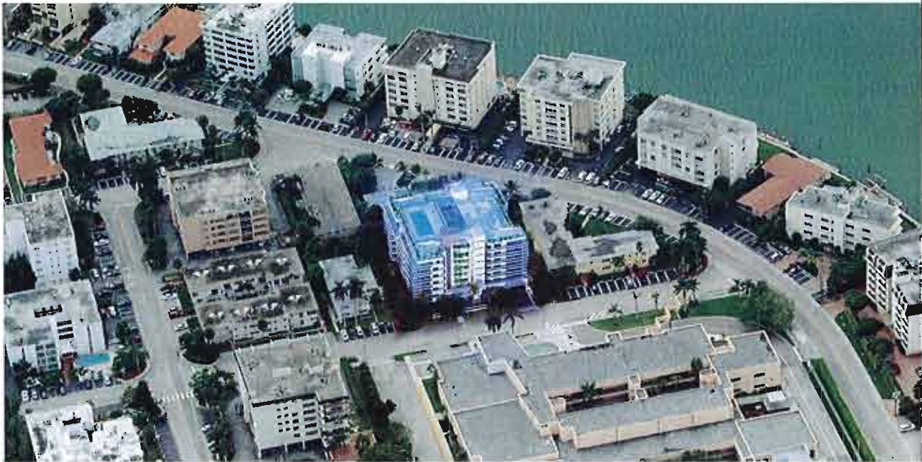
AERIAL VIEW FROM NORTHEAST
