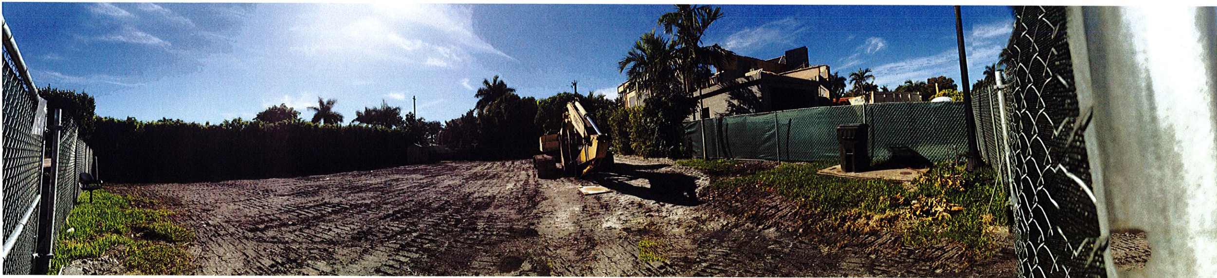
5.SOUTH VIEW TOWARDS SITE SHOWING EAST, WEST, AND REAR ADJACENT PROPERTIES
