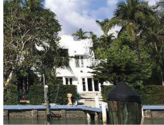
CS-02 LOT 25 REAR EXISTING VIEW (EAST)
