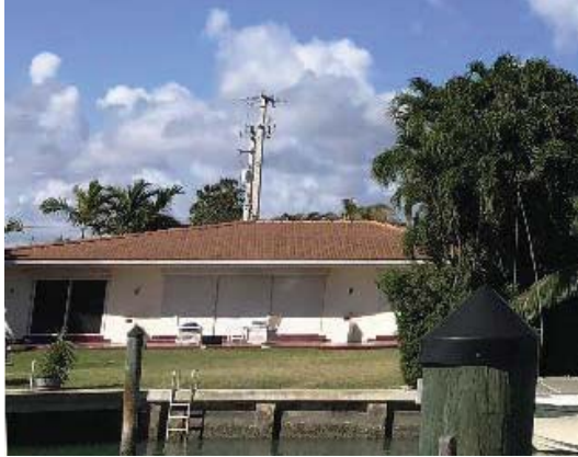
CS-02 LOT 23 REAR EXISTING VIEW (EAST)
