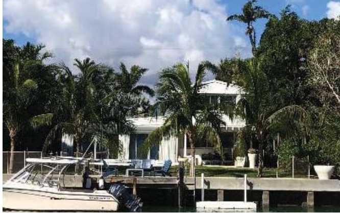
CS-02 LOT 24 REAR EXISTING VIEW (EAST)
