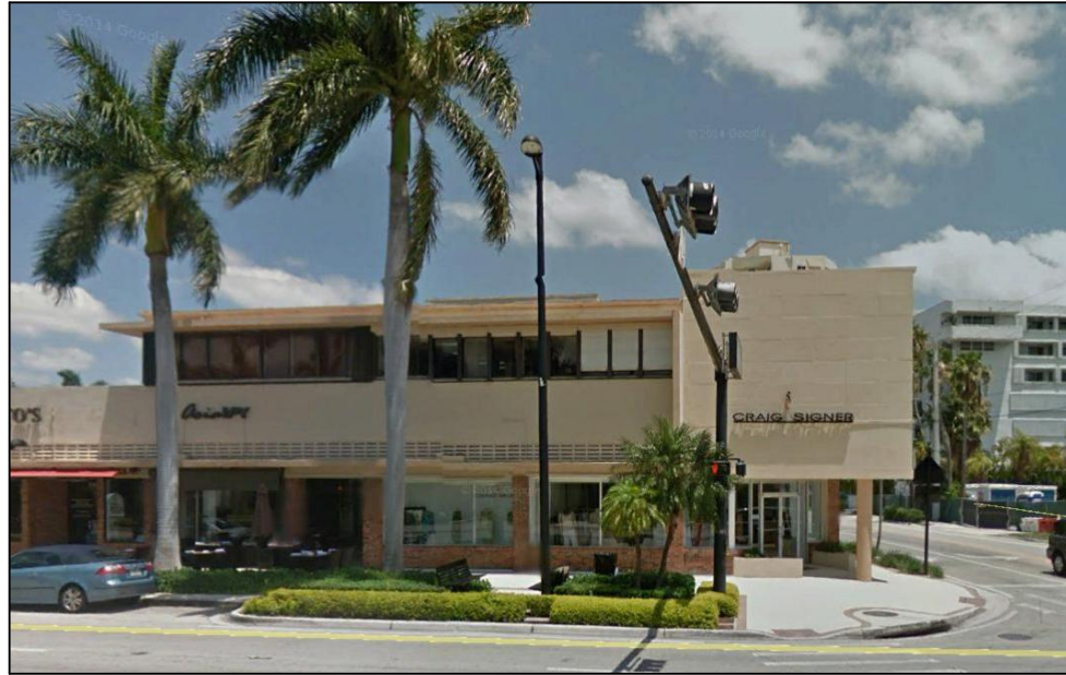
OFFICE, BUSINESS DISTRICT FLUM: COMMERCIAL 1 STORY
