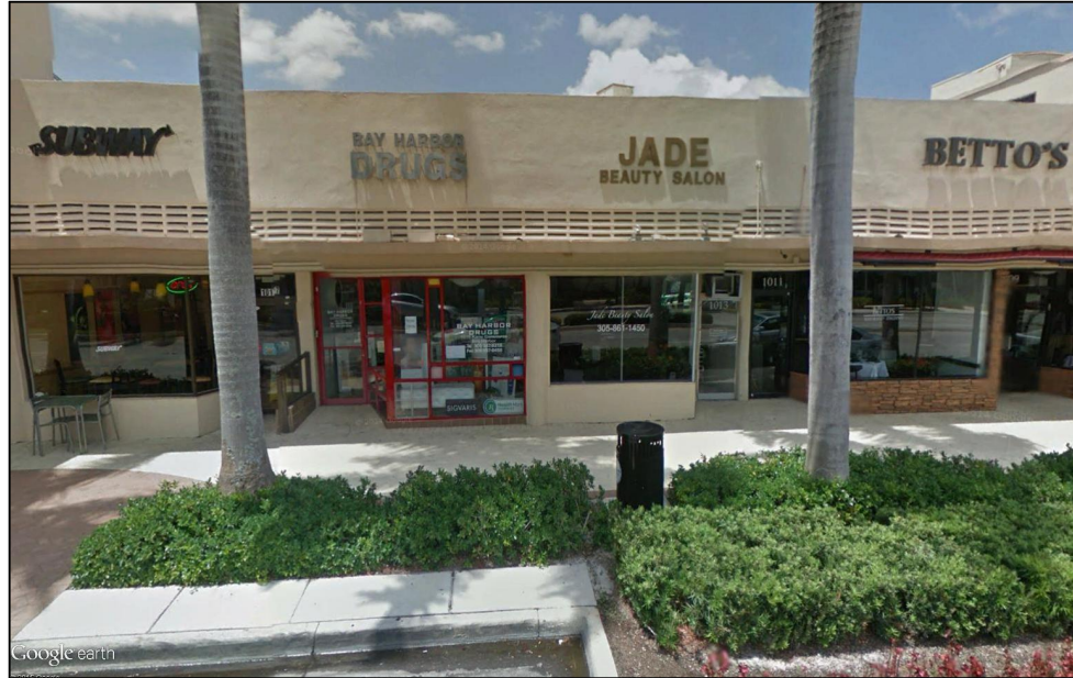
OFFICE, BUSINESS DISTRICT FLUM: COMMERCIAL 1 STORY
