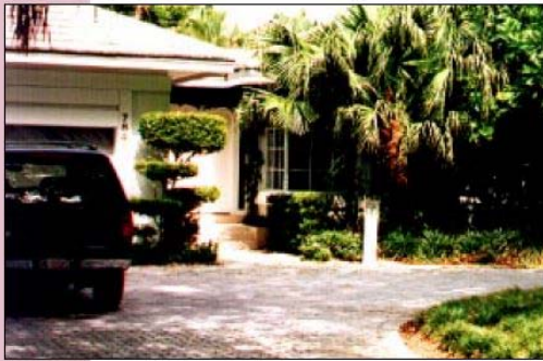
Concrete unit pavers add texture and color to this driveway.
