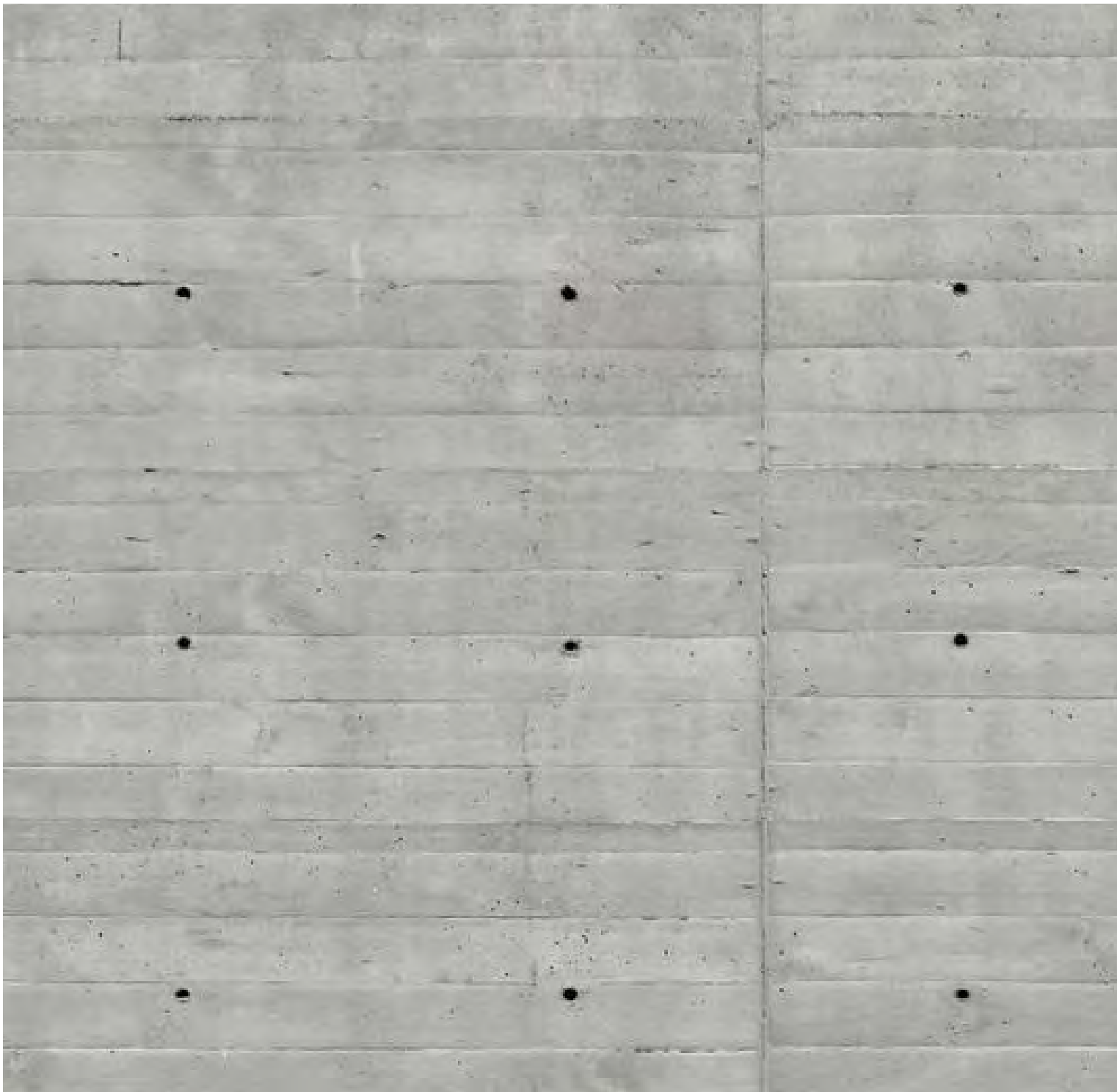
CONCRETE Exterior Balcony Projections
