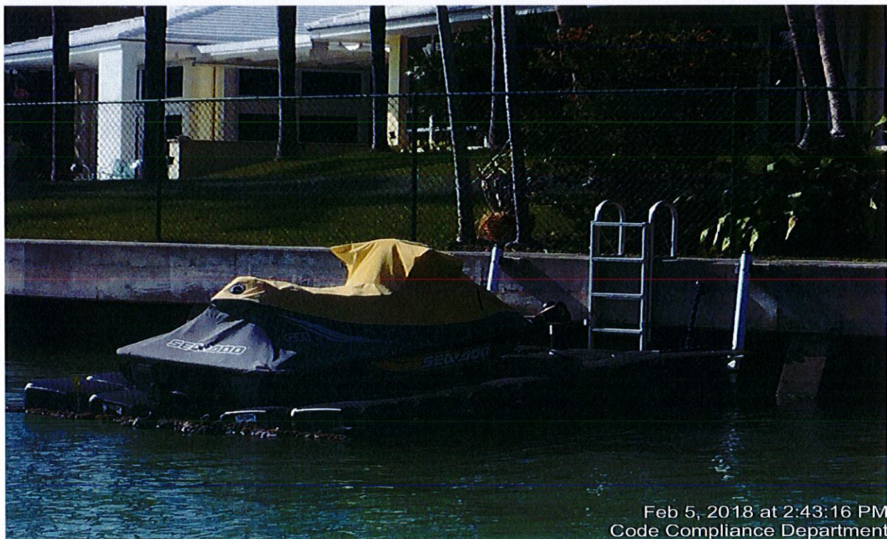
14- 9405 East Broadview Drive- Floating dock attached to the seawall.
