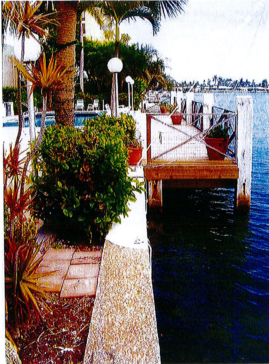
Photo 598: Property 147 – Looking east from west property line. Note concrete overlay on the Chattahoochee stone.
