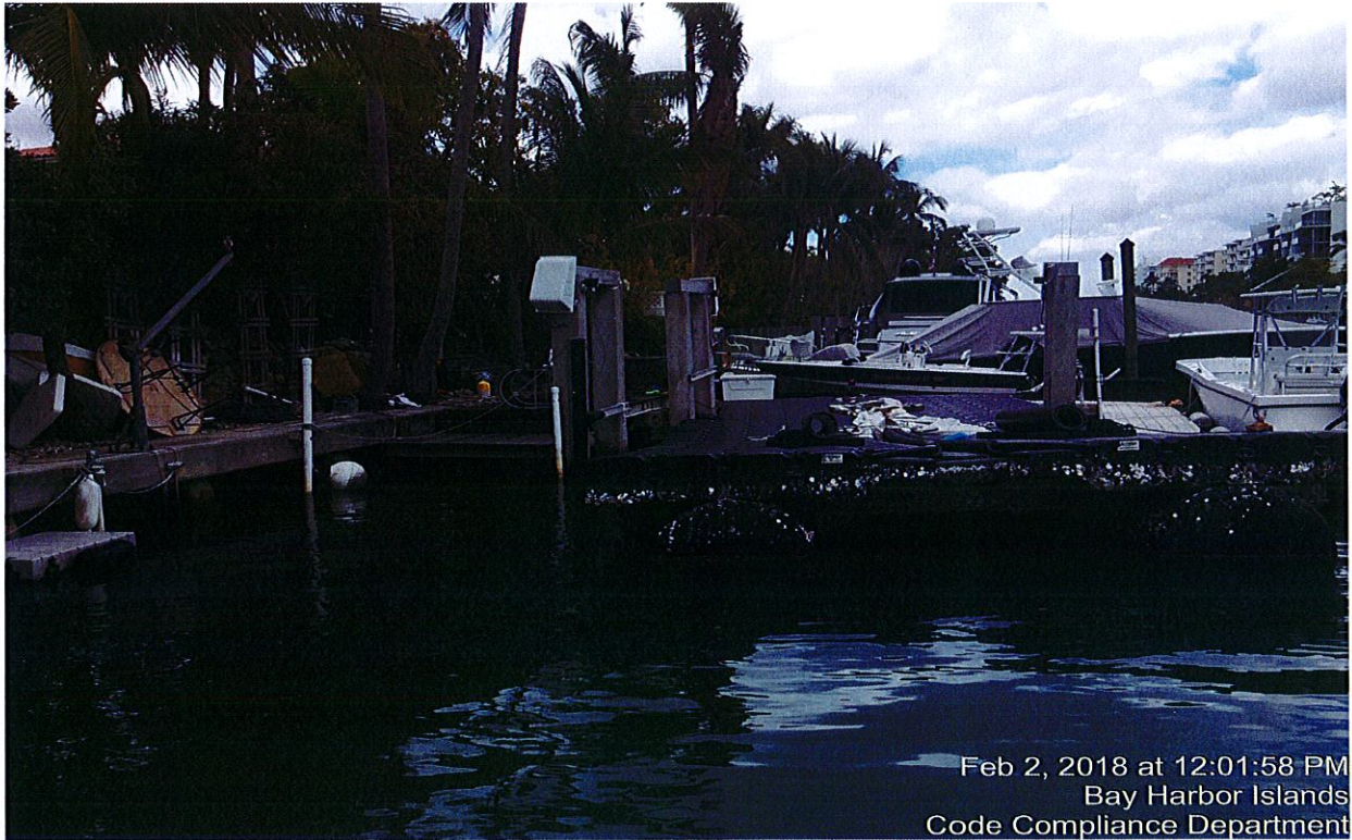
3- 9721 East Broadview Drive- Floating dock attached to the seawall.
