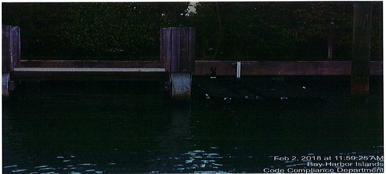
1- 9601 East Broadview Drive- Floating dock attached to the seawall.
