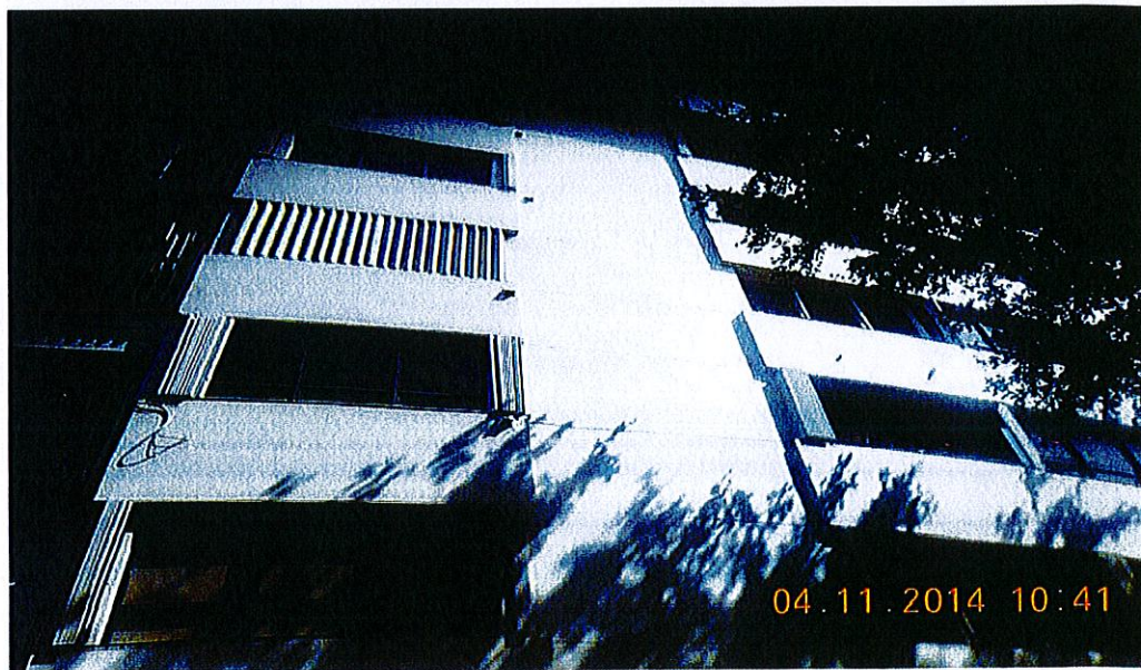
South side of the property- No violations observed.
