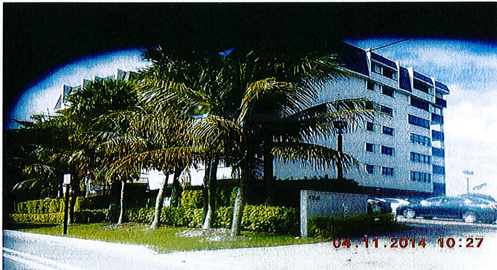
Street view of the property – No violations observed.
