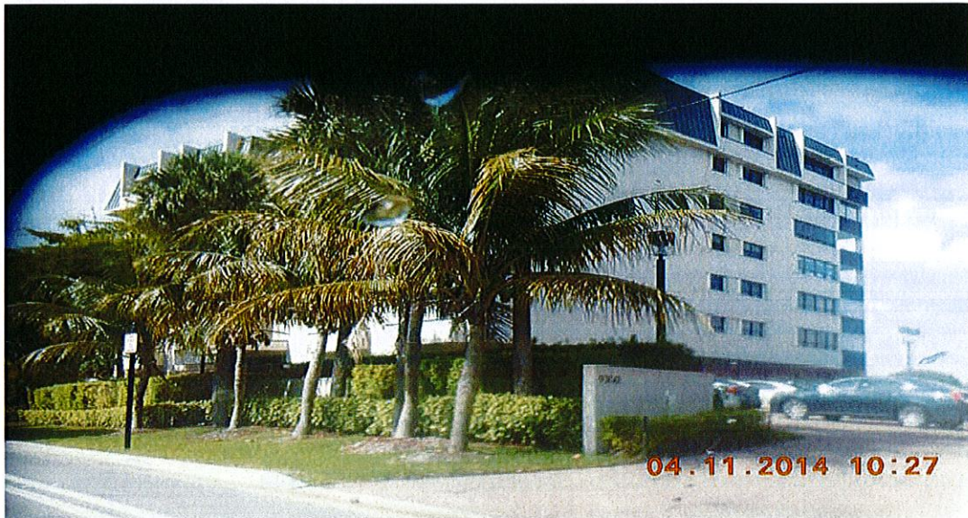
Street view of the property – No violations observed.
