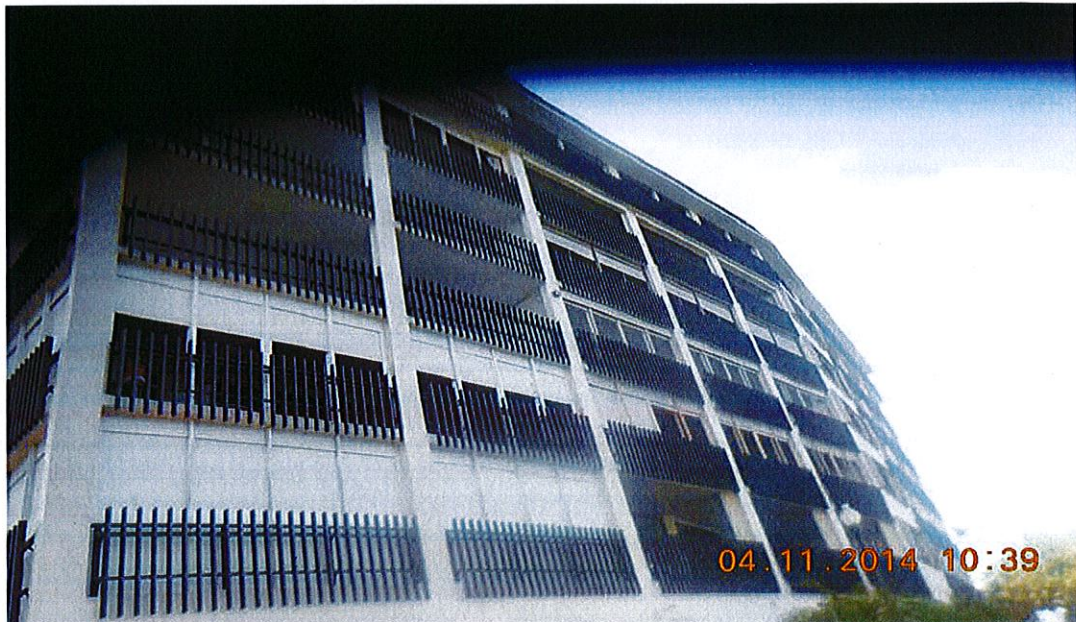
East side of the property- No violations observed.
