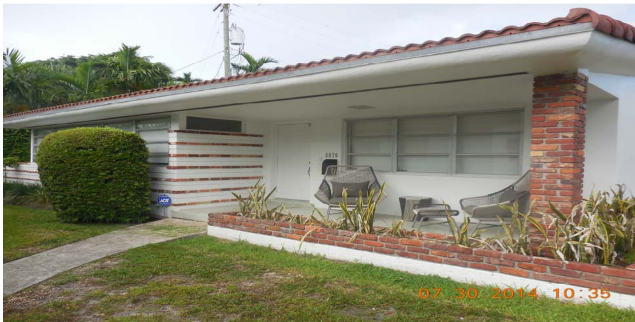
Building 9976- No violations observed.
