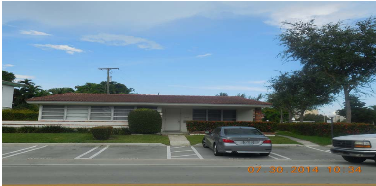
Building 9970- No violations observed.
