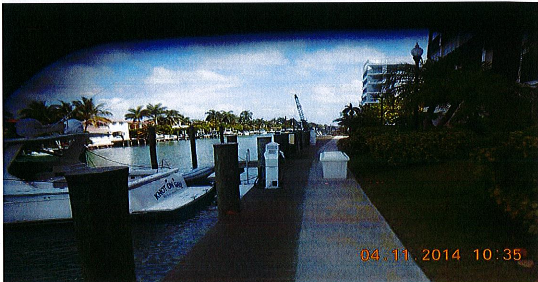
Dock - No violations observed.
