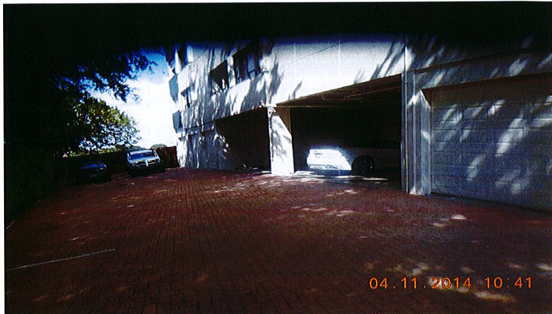
South side parking area- No violations observed.
