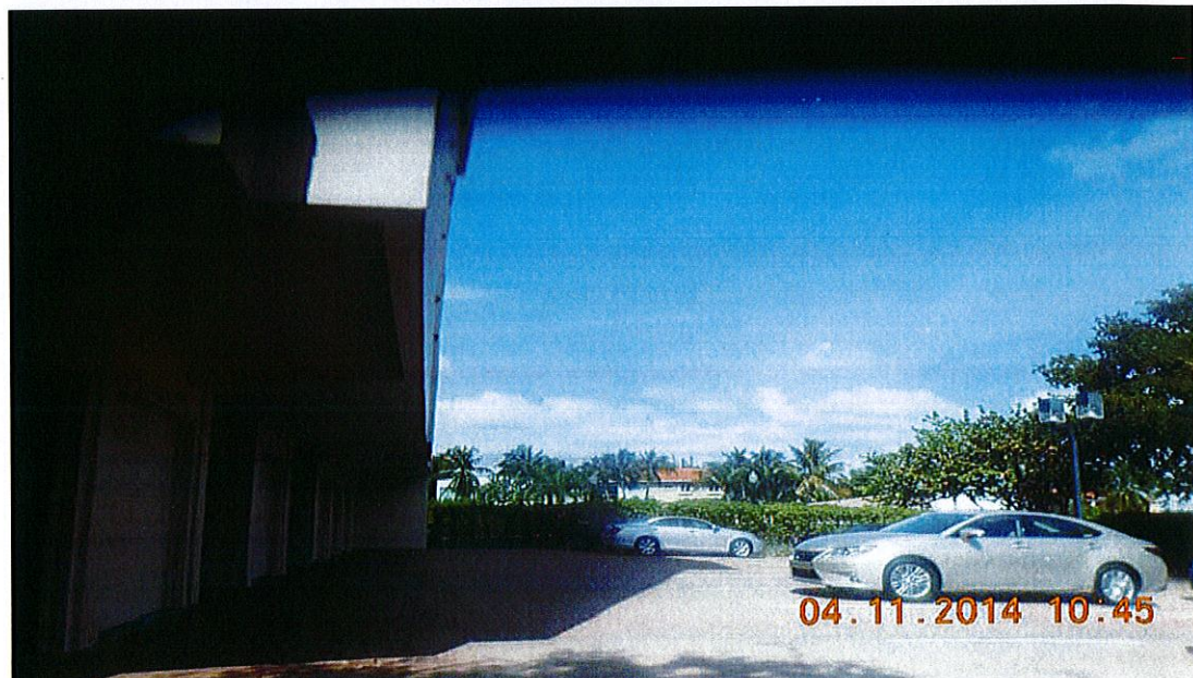
North side parking area- No violations observed.
