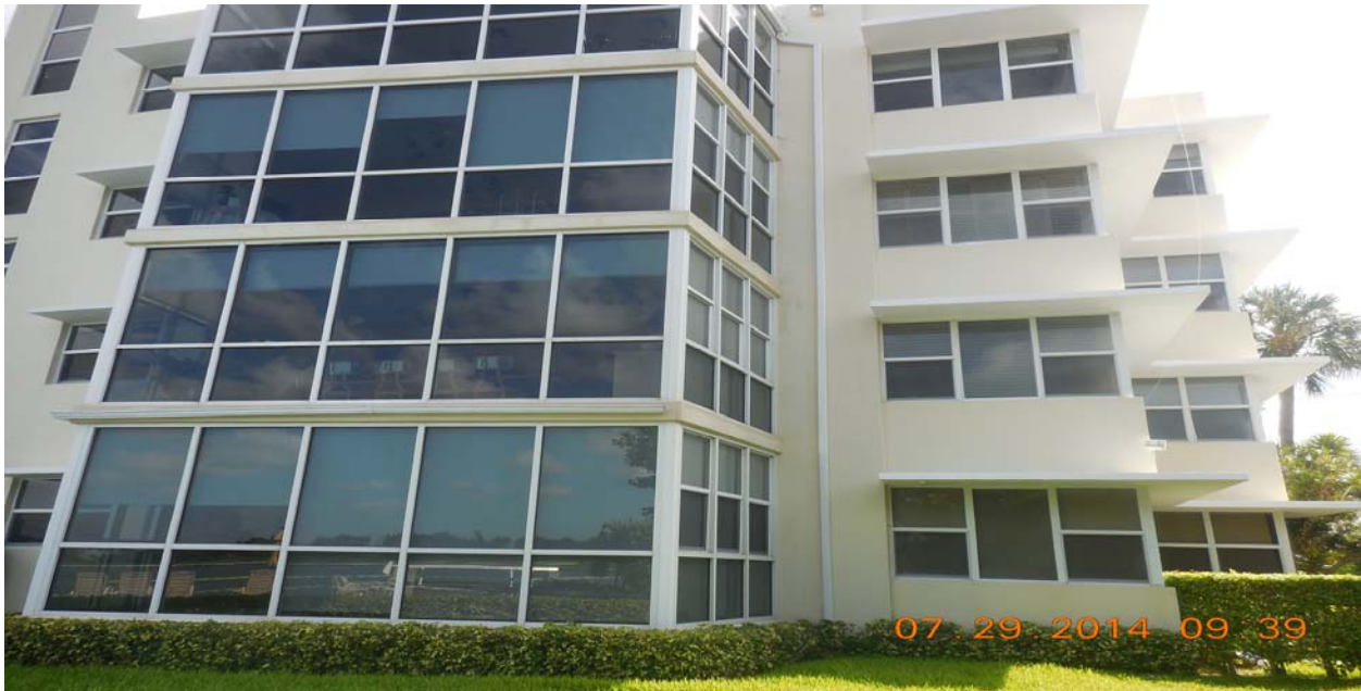
View of the south side of the property- No violations observed.
