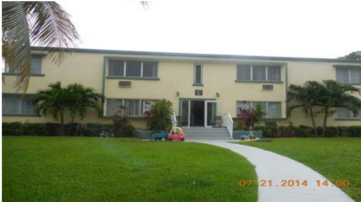
View of 10270 building- No violations observed.
