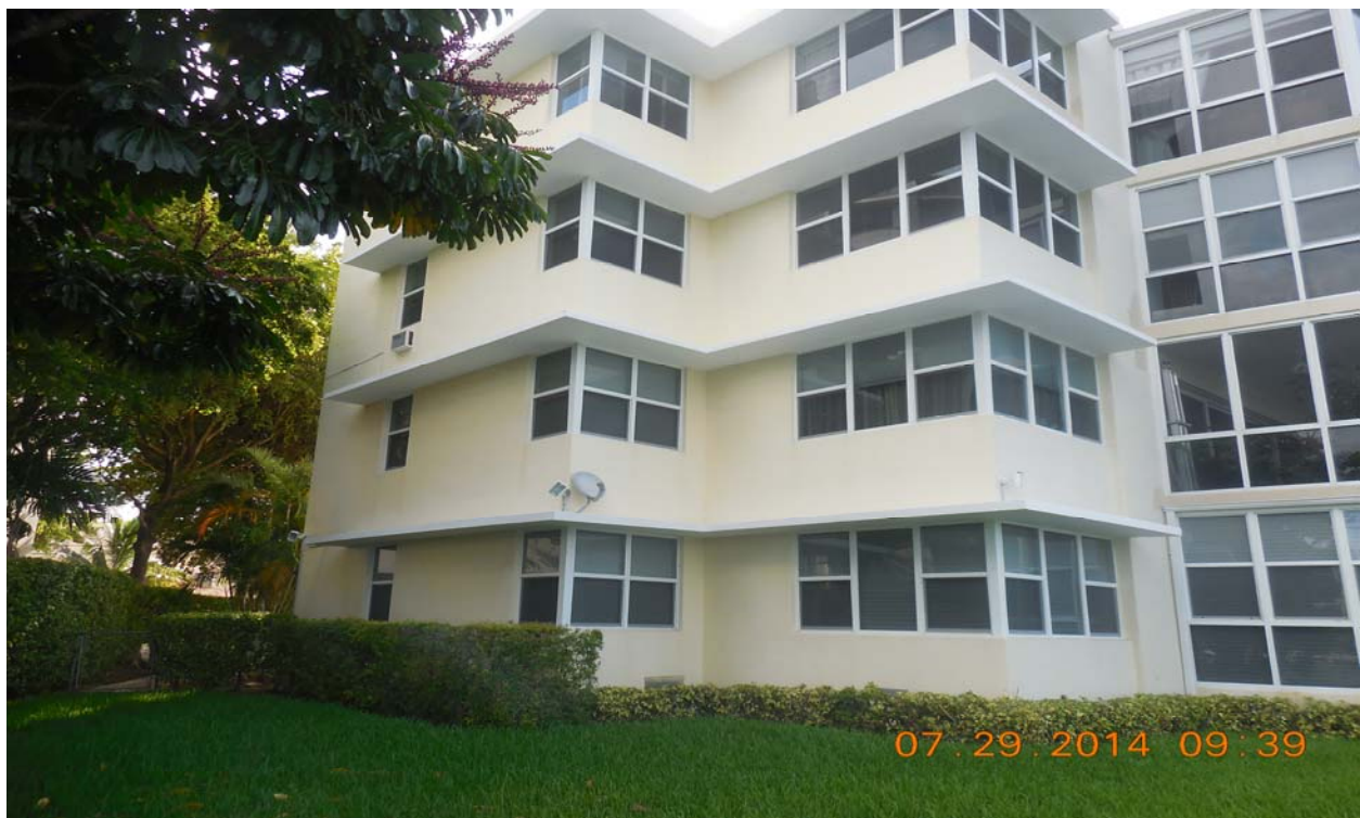
View of the north side of the property- No violations observed.
