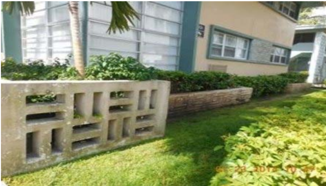
View of the property from 98 street- Planters located in front of the property are dirty and need to be pressure cleaned.
