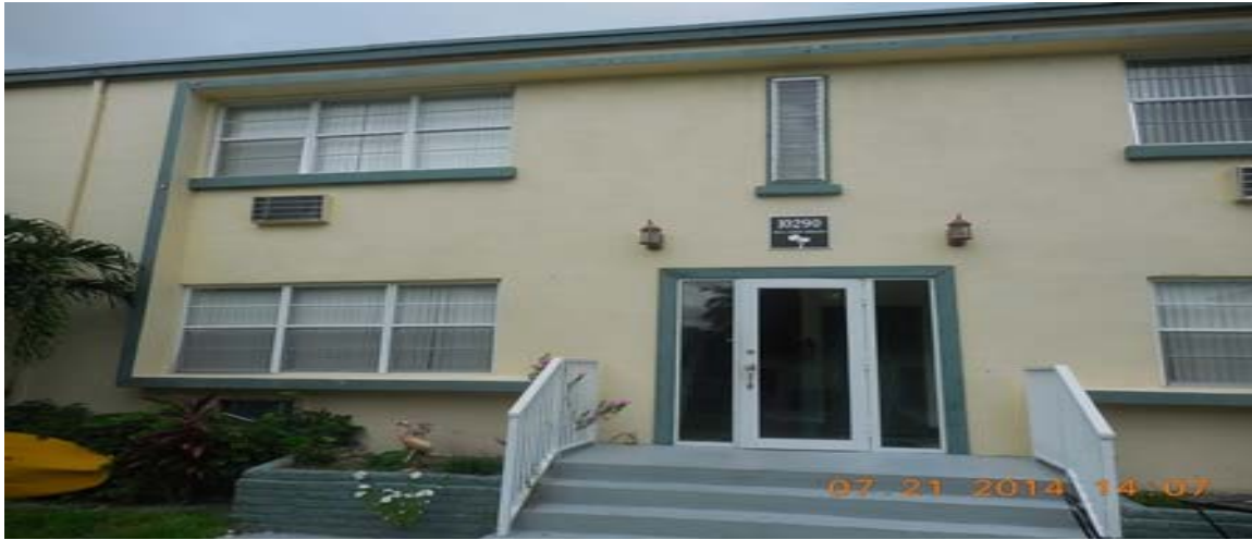
View of building 10290- No violation observed.
