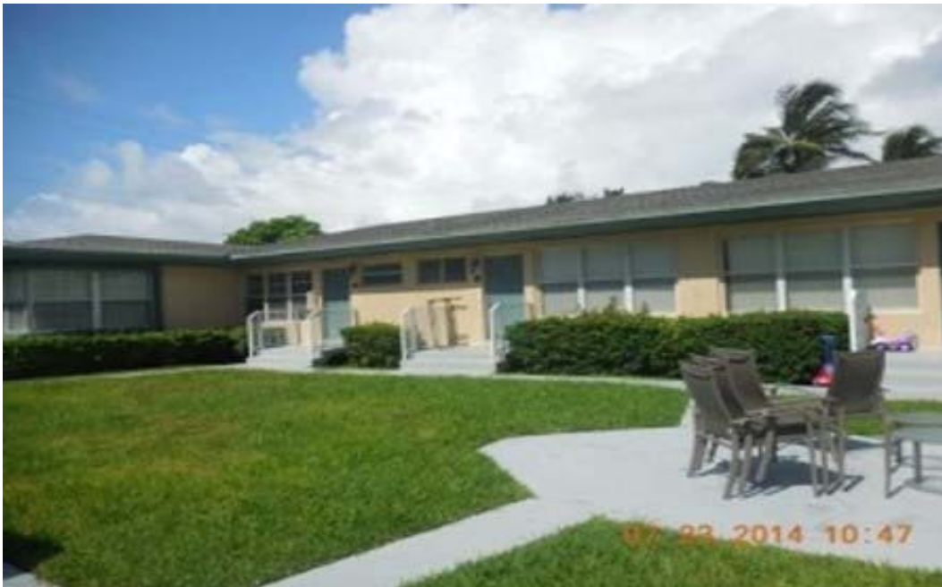
Southeast view of the property- No violation(s) observed.
