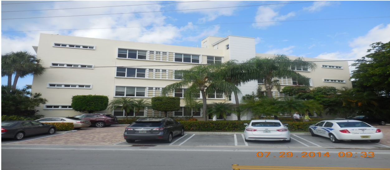
View of the property from West Bay Harbor Drive- No violations observed.
