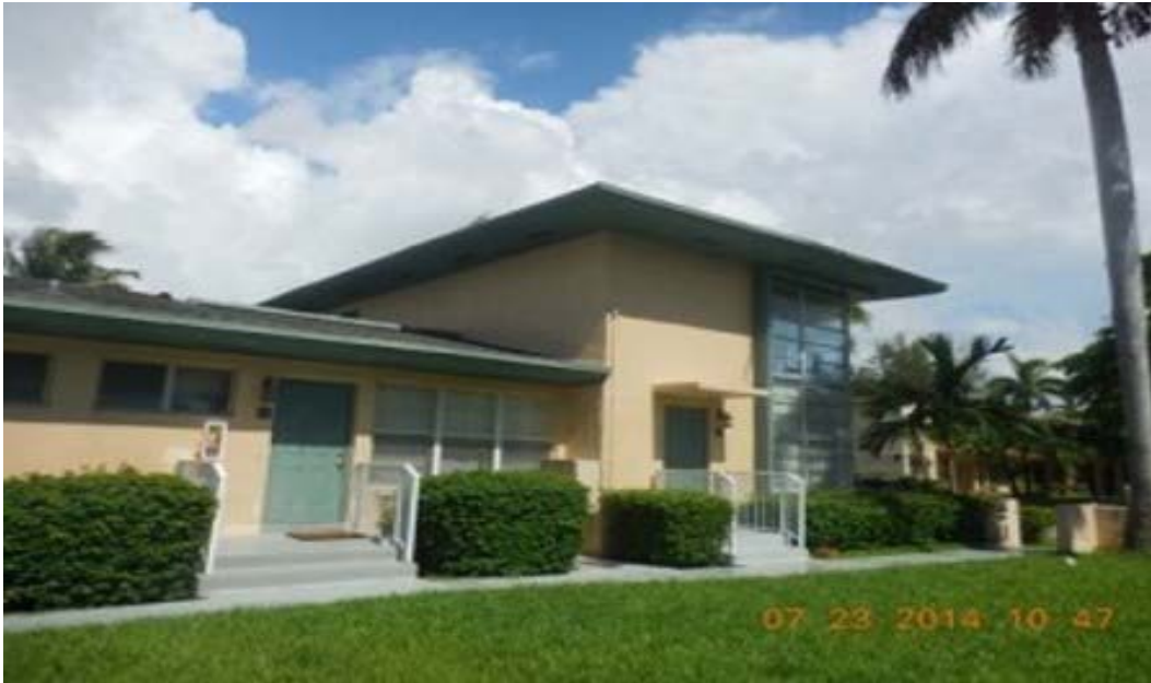
Front view of the property- No violation(s) observed.
