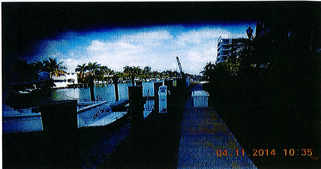
Dock - No violations observed.
