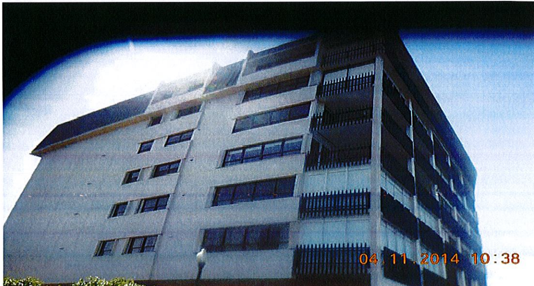
North side of the property – No violations observed.
