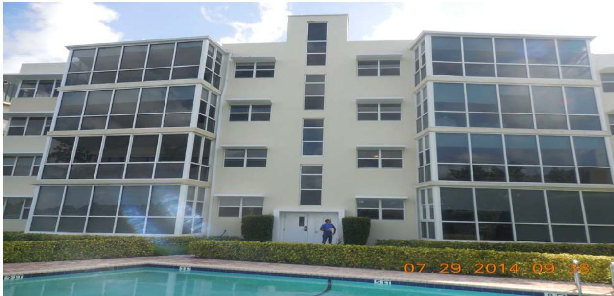
View of the property from the waterside- No violations observed.
