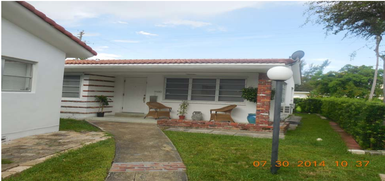
Building 9980- No violations observed.
