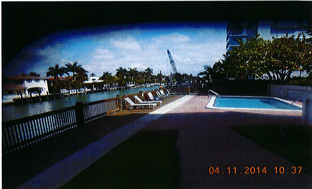
Pool area- No violations observed.
