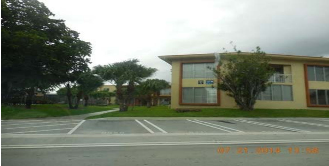
View of the property from East Bay Harbor Drive
