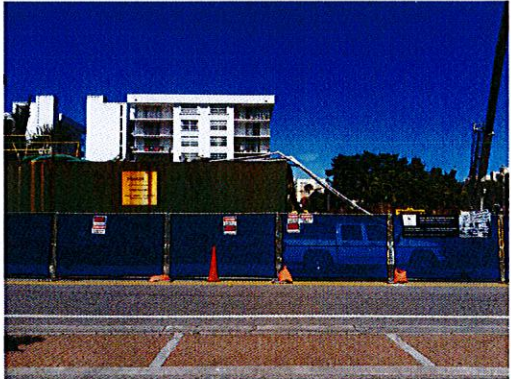
EXIST. EAST PROPERTY NEIGHBOR (UNDER CONSTRUCTION)
