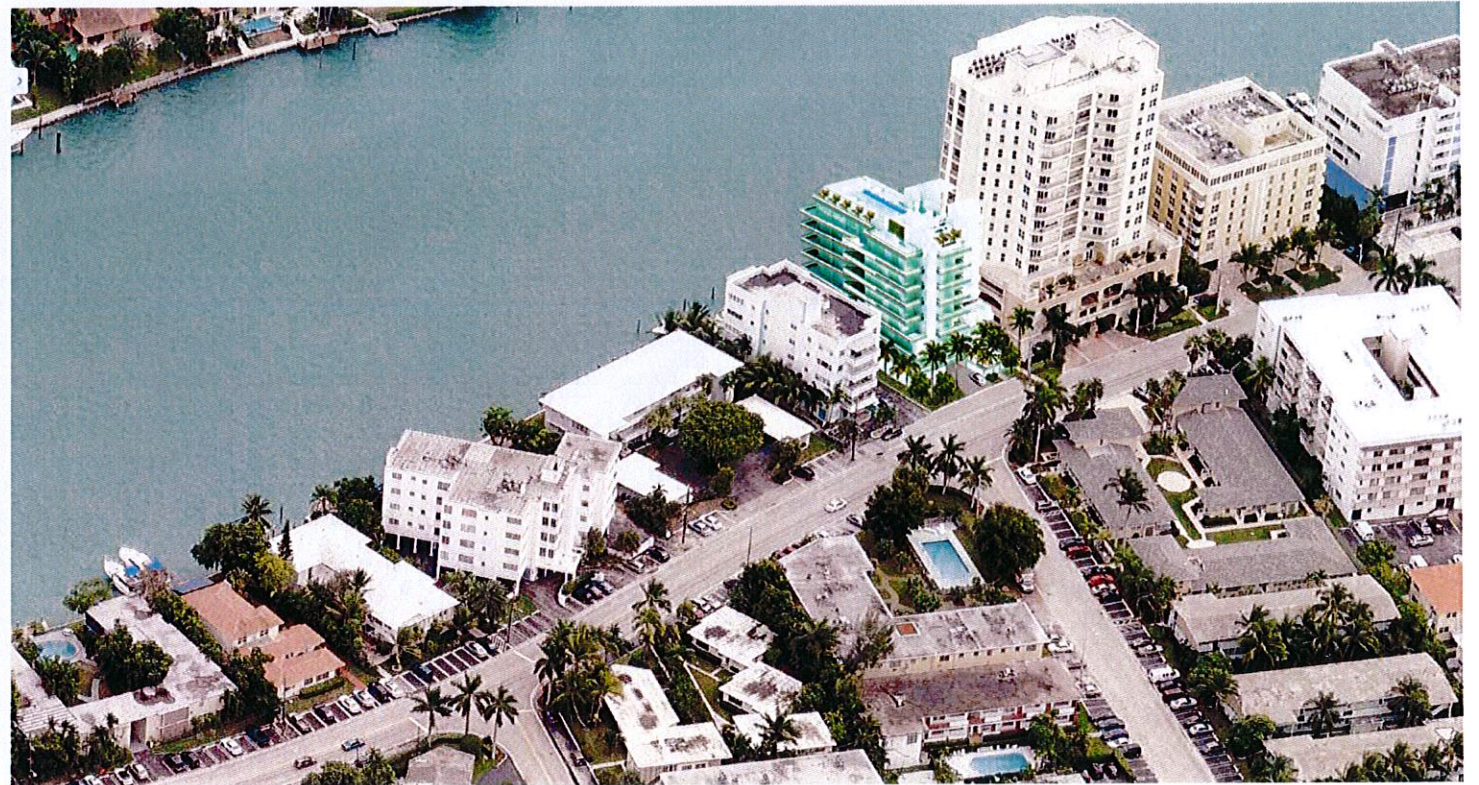
AERIAL VIEW FROM NW
